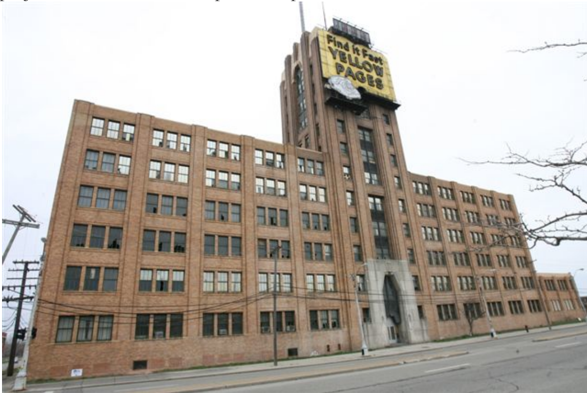
Built in 1929 and 1930, the 12-story Art Deco-style Michigan Bell and Western Electric Warehouse is located at 882 Oakman Blvd., between Detroit and Highland Park.
